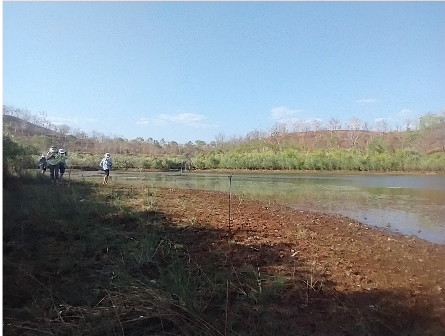
Copperfield Dam, Pine Creek © Scott Roberts
